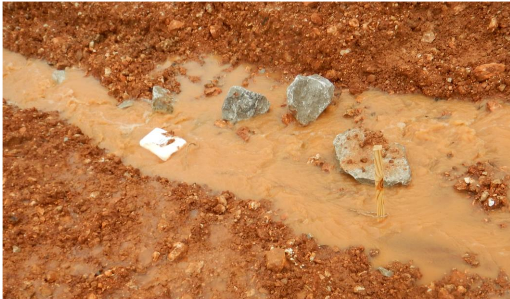
Figure 2.2: Photograph of the APS 703d type Floc Log roped around a stake. Photo taken by Bryan Signorelli (AHTD) on June 18, 2015.
